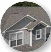
Roofing and Ventilation
